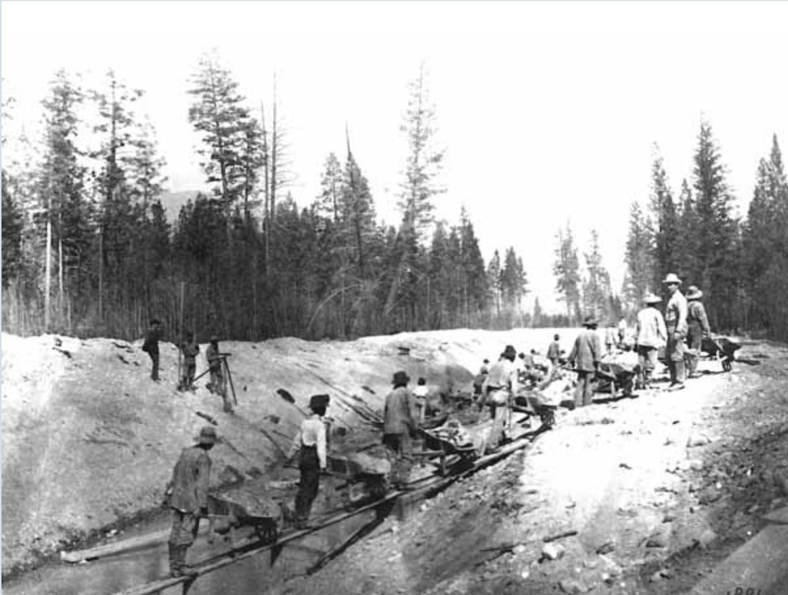
FIG 3-1 Chinese workers building the CPR main line, 1884. Library and Archives Canada, C-6686 B.
