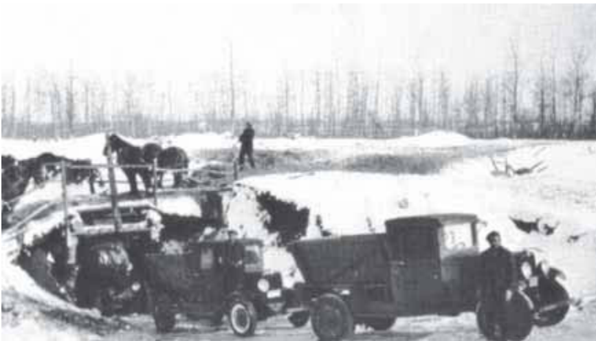
Road Construction, Elk Island National Park, 1930s
