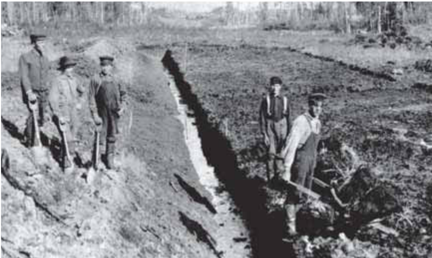
Grand Trunk Pacific Railway construction in the Tofield area. c. 1906 Construction work provided supplementary employment for many attempting to settle in the inner reaches of the Beaver Hills.
