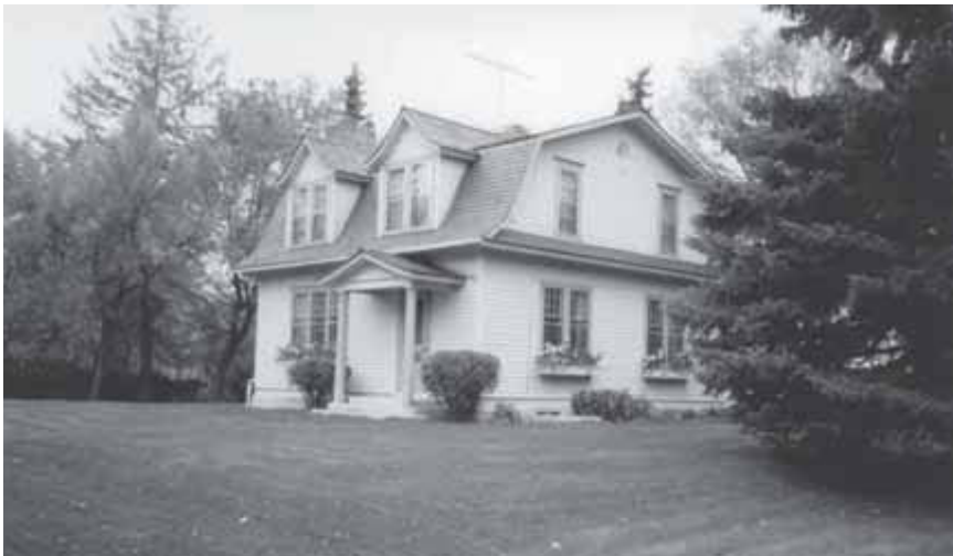
Restored Superintendent's Residence, Elk Island National Park, 1985 The growing community interest in preserving the pioneer heritage extended to long serving public buildings.
