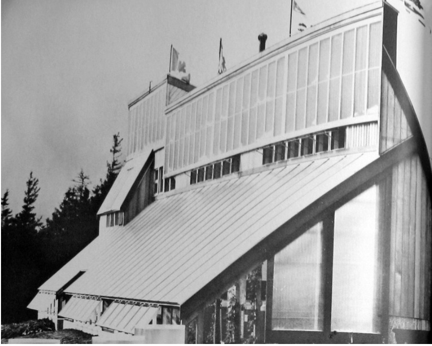
7.3 The PEI Ark viewed from the south. The greenhouse is in the right foreground and the living area in the left background. Source: An ARK for Prince Edward Island .
